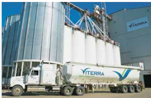
Feed processing plant at Sherwood Park, Alberta.
